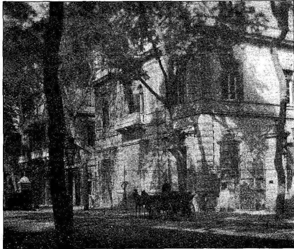
Y.W.C.A. HOME. FRONT VIEW, THIRD FLOOR.
